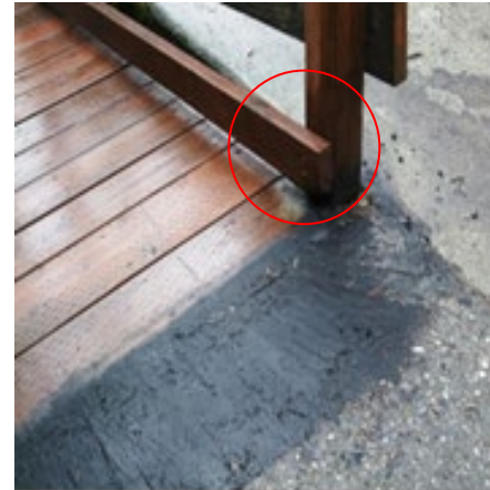
Ramp Edge Guard (red circle)
