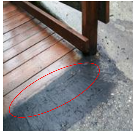
Asphalt Cold Patch is Used to Reduce This Threshold Edge (red circle)
